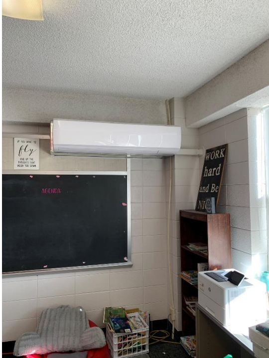
Ductless Mini-split Indoor Unit
