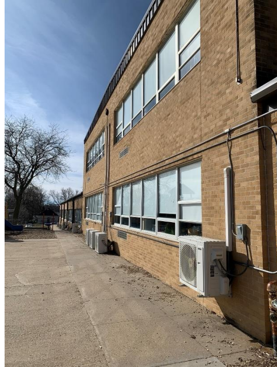
Ductless Mini-split Outdoor Units
