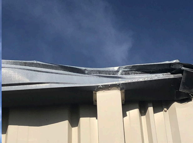
Gutter damage
