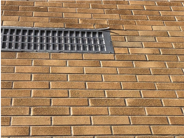
Deteriorating sealant
