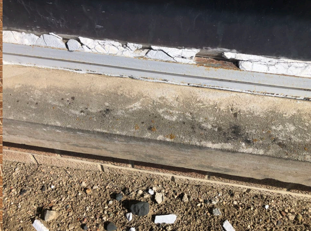
Sealant is no longer flexible
