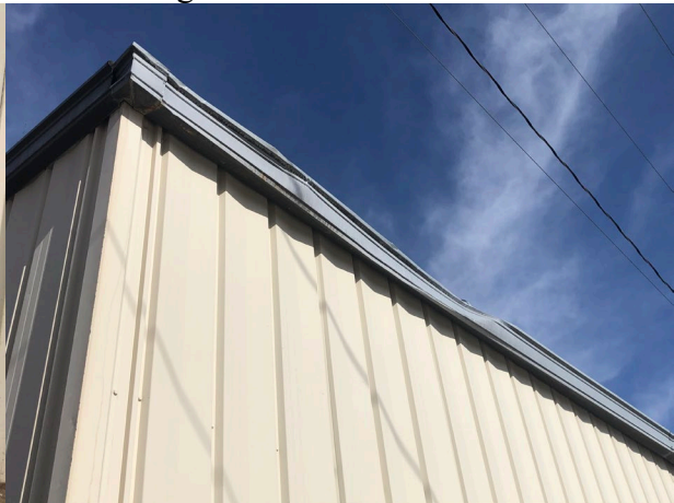
Gutter damage
