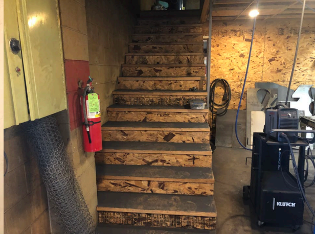
Metals shop mezzanine stair lacks guard and hand rails.
