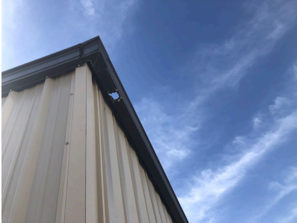
Missing downspout
