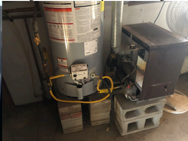
Water heater and space heater are exposed in the office. The smell of gas/exhaust evident
