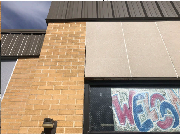
Sealant missing
