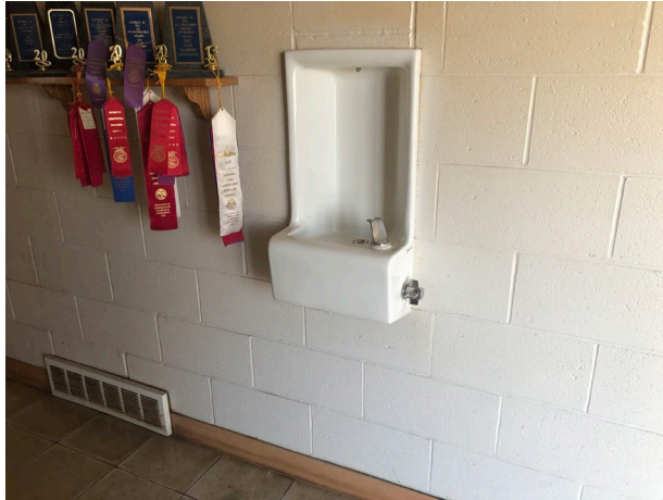
No knee and toe clearance at water fountain Fountain should also be a high/low model
