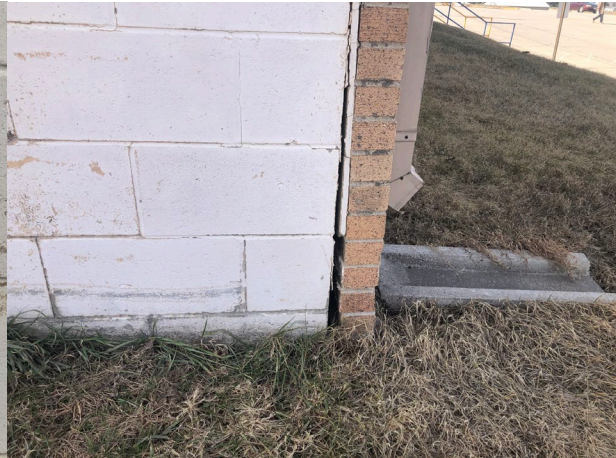
Movement of CMU/brick veneer
